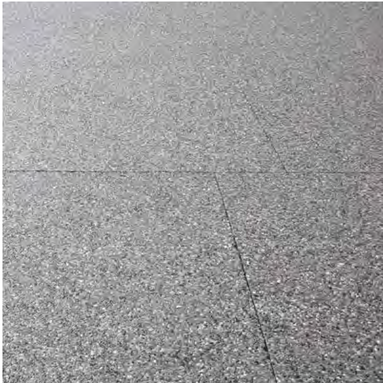
CONCRETE TYPE 1: EXPOSED AGGREGATE
