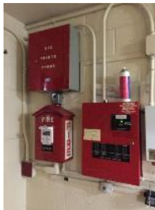
Fire Alarm Control Panel
