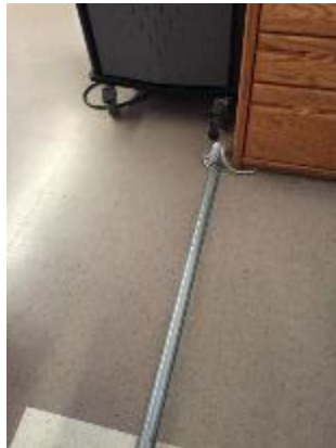
Floor Mounted Raceway
