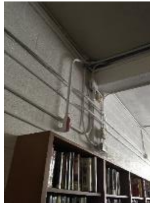
Example Of Surface Conduit
