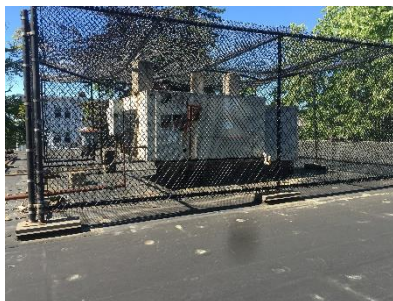
RTU w/ Patio blocks Holding up Fence Roof
