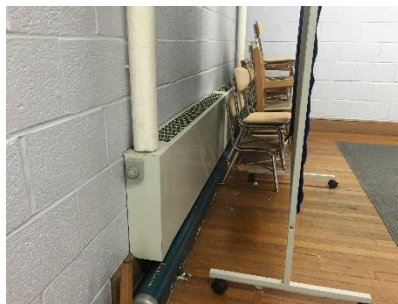
HW Baseboard w/ Self-Contained Valve
