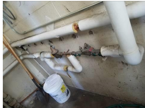
Backflow Preventer for Make-up Water
