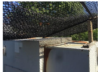
Chainlink Enc. Roof Collapsed on RTU
