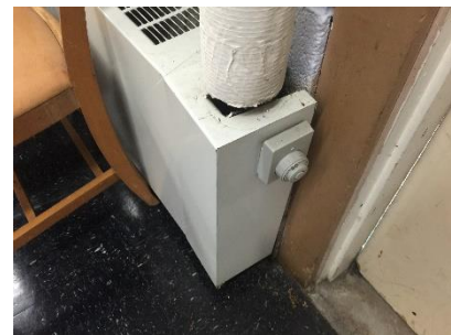
Self-contained Valve Adjustment
