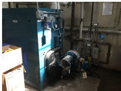
Gas-Fired Boiler
