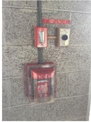
Annunciator and Pull Station
