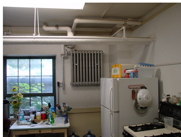
Existing Wall-hung Radiator
