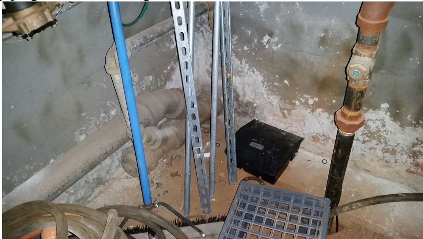
Existing 4" Sanitary Pipe Exit Building above Basement Floor Slab
