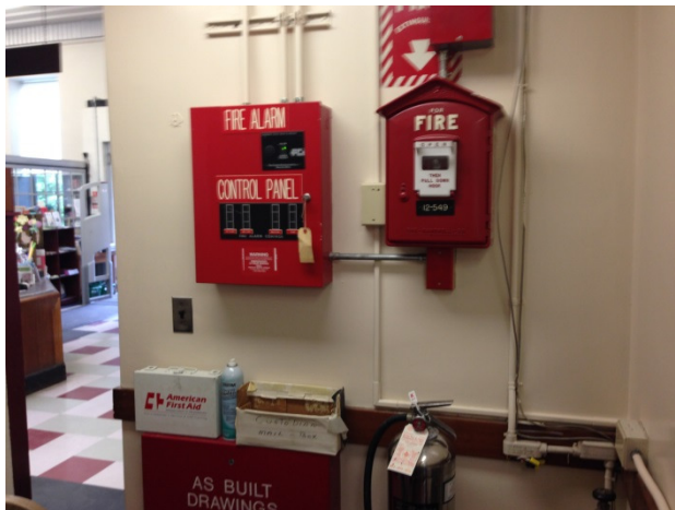
Existing Fire Alarm Control Panel
