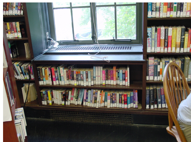
Existing Enclosed Radiator Under Window
