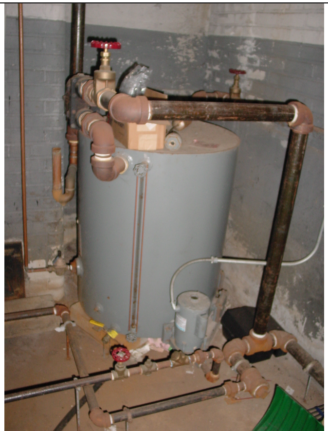
Existing Condensate Receiver
