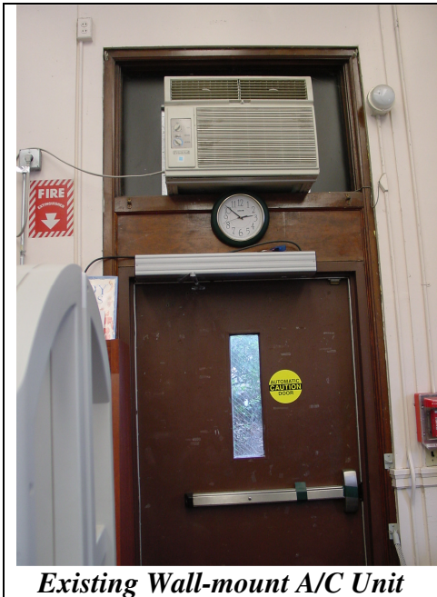
Existing Window-mount A/C unit in a Crowded Room
