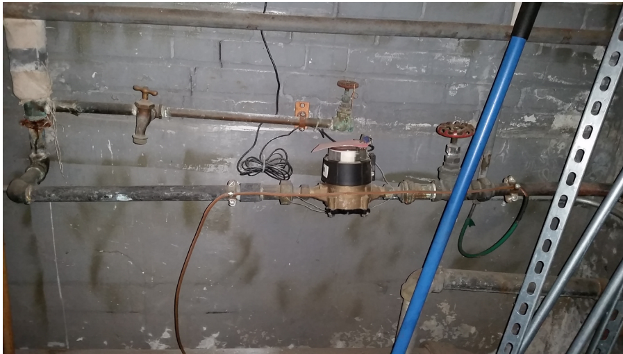
Existing Water Service and Water Meter
