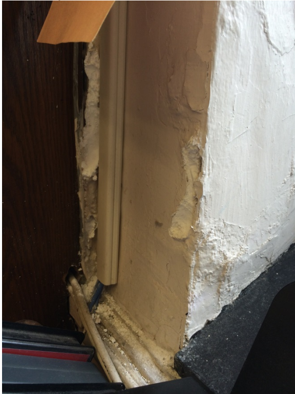
DETERIORATED PLASTER AT WINDOW JAMB
