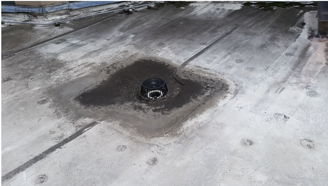
Existing Roof Drain
