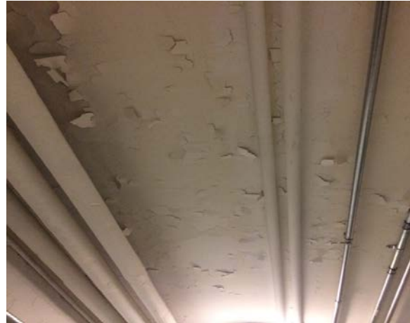
PEELING PAINT IN BASEMENT
