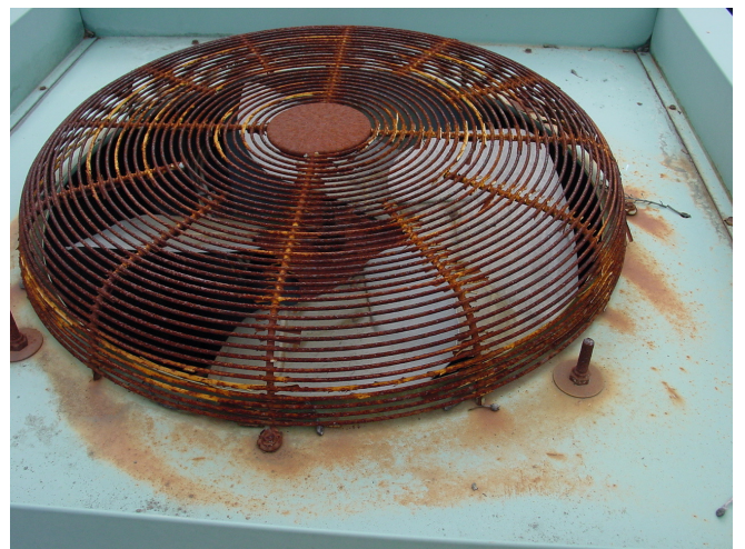
Rust on Existing Rooftop Condenser
