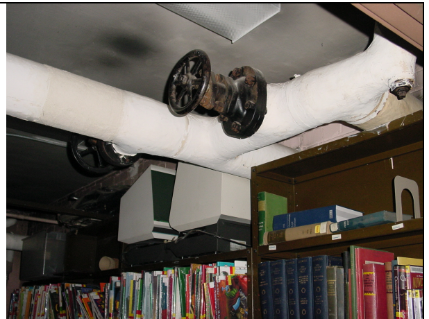
Old Insulation on Existing Steam Pipes
