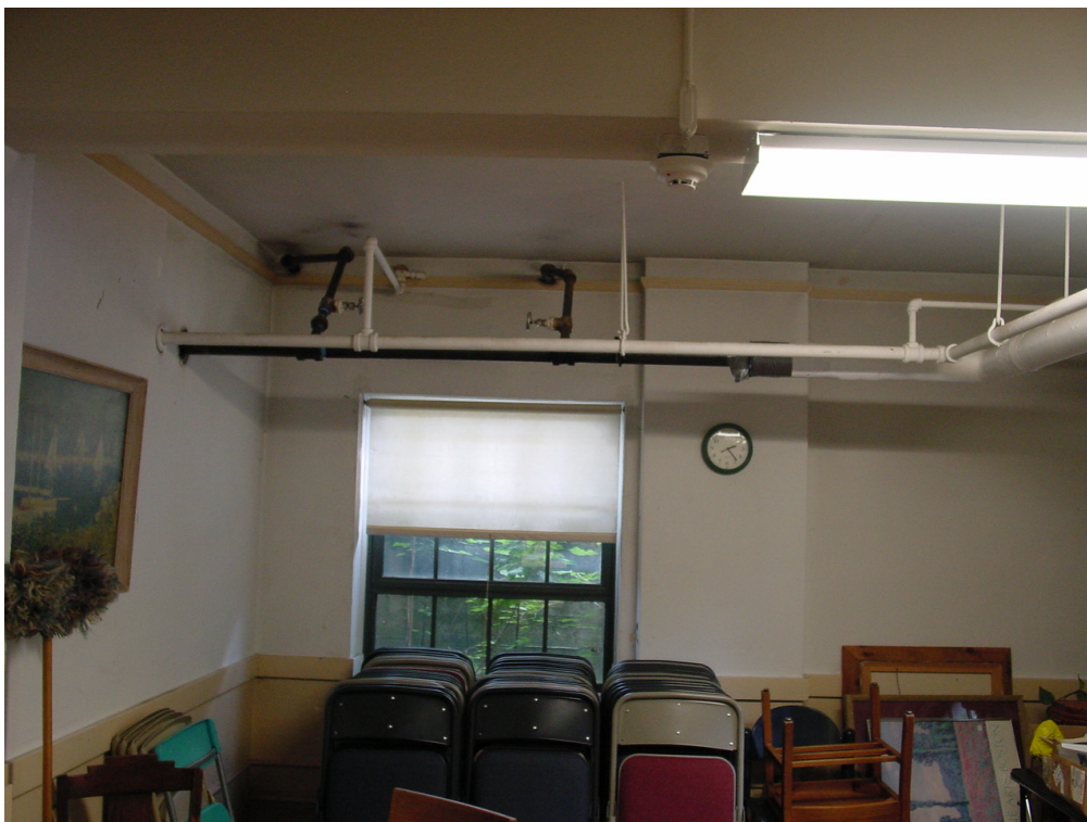
Existing Steam and Condensate Pipes Running through Occupied Space
